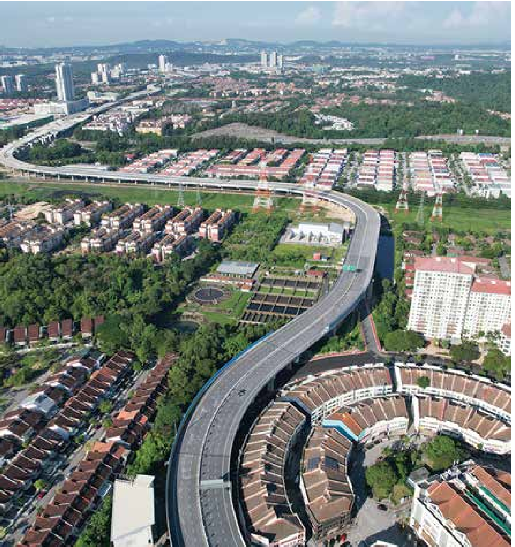
Location: Damansara Perdana, Damansara-Shah Alam Elevated Expressway.
