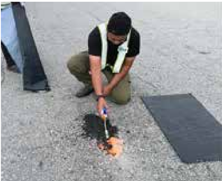
Carpet patching is one of our effort towards zero pothole target.
