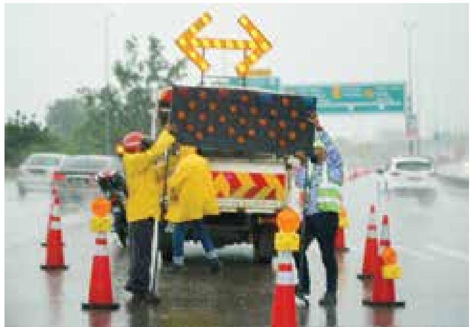
Setting up traffic management for emergency situation.
