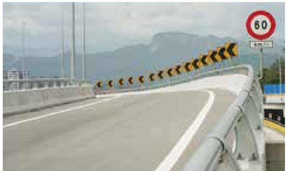
Clearly visible warning signs.
