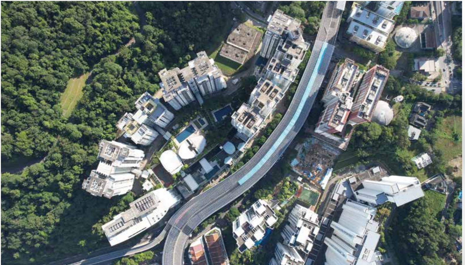
➤ DASH Highway: Designed with Communities, Environment and Safety in mind.
