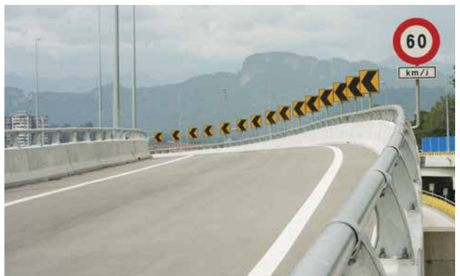
Clearly visible warning signs.
