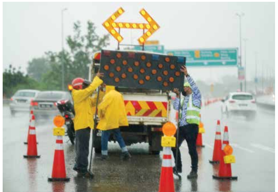
Setting up traffic management for emergency situation.
