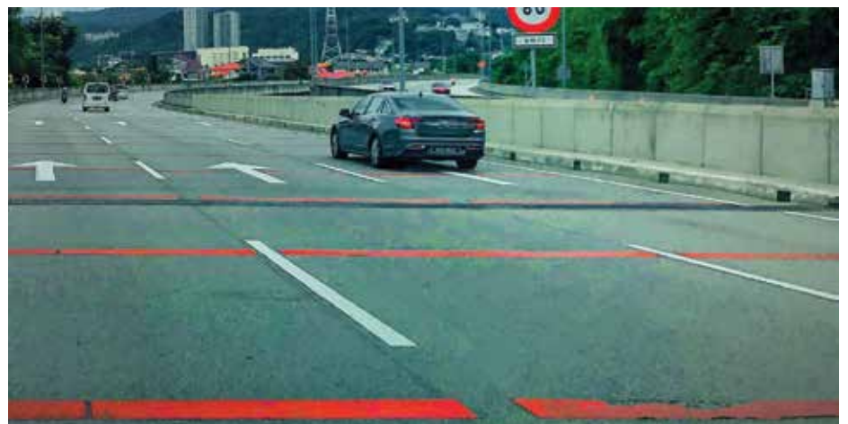
Road lane markings and rumble strips.
