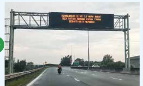
Notification of accident to road users.
