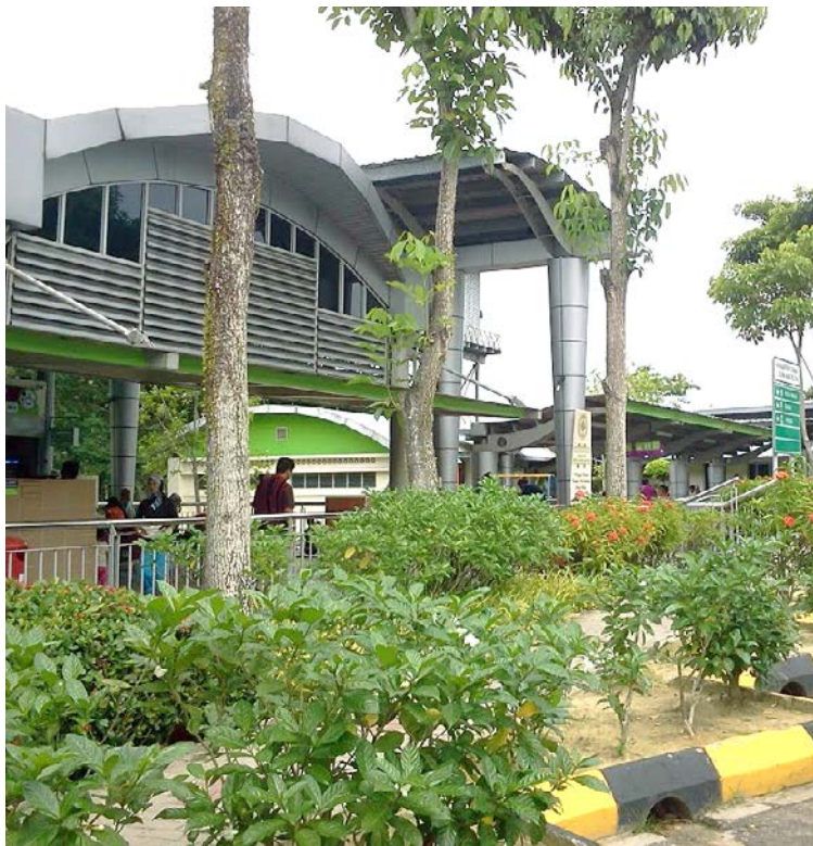
RSA Elmina Before Rejuvenation
