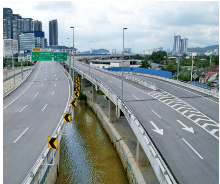
→ The structure splits the road into separate carriageways with an opened penetrating gap in the middle that allows sunlight to reach the river life.
