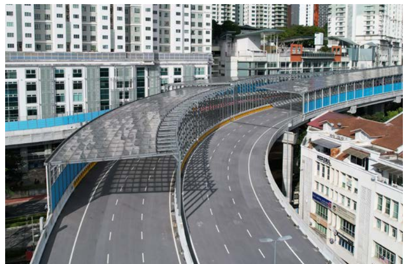
→ We mitigate the noise pollution associated with our highway operations by conducting annual noise monitoring and the installation of noise barriers.
