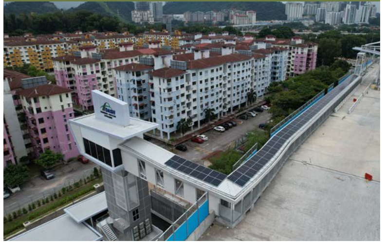
➡ Rooftop solar PV installed at Kota Damansara Toll Plaza, DASH.
