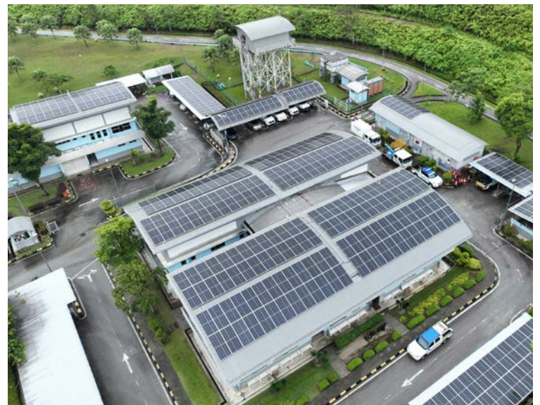
➔ Solar panel installed at Plaza Toll Elmina, GCE.
