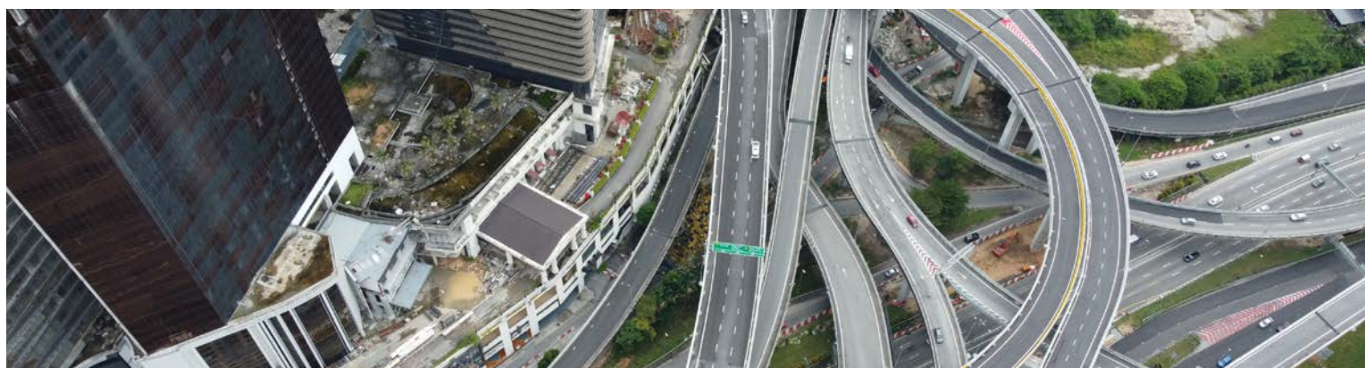
→ Penchala Interchange, Damansara-Shah Alam Elevated Expressway
