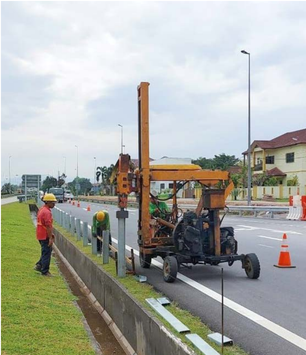
→ A contractor carrying out maintenance works.
