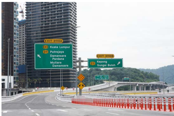
➔ Flexible safety post, reflective safety signage and road and directional signboard at DASH Highway.
