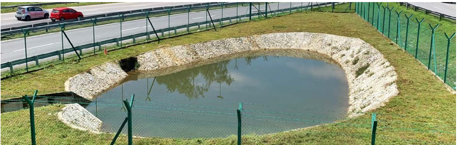
Retention pond at GCE that is designed to store excess rainwater or runoff from surrounding areas, thereby reducing the risk of flooding.
