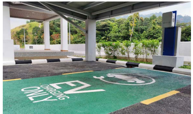
→ Our EV Charging Station at Toll Plaza Bukit Teratai Lay-by, SUKE.
