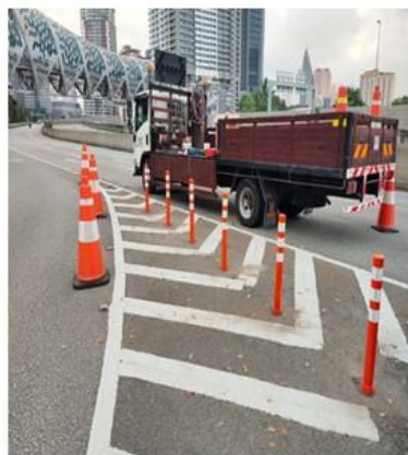
Reinstatement and Cleaning of Flexible Poles at SILK, AKLEH & LKSA
