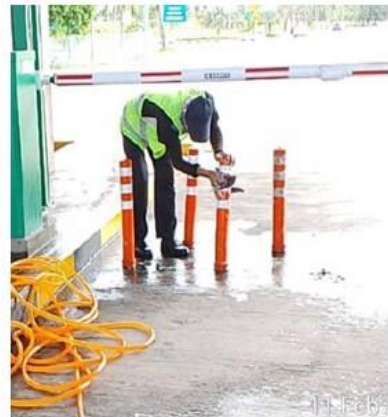
Reinstatement and Cleaning of Flexible Poles at SILK, AKLEH & LKSA
