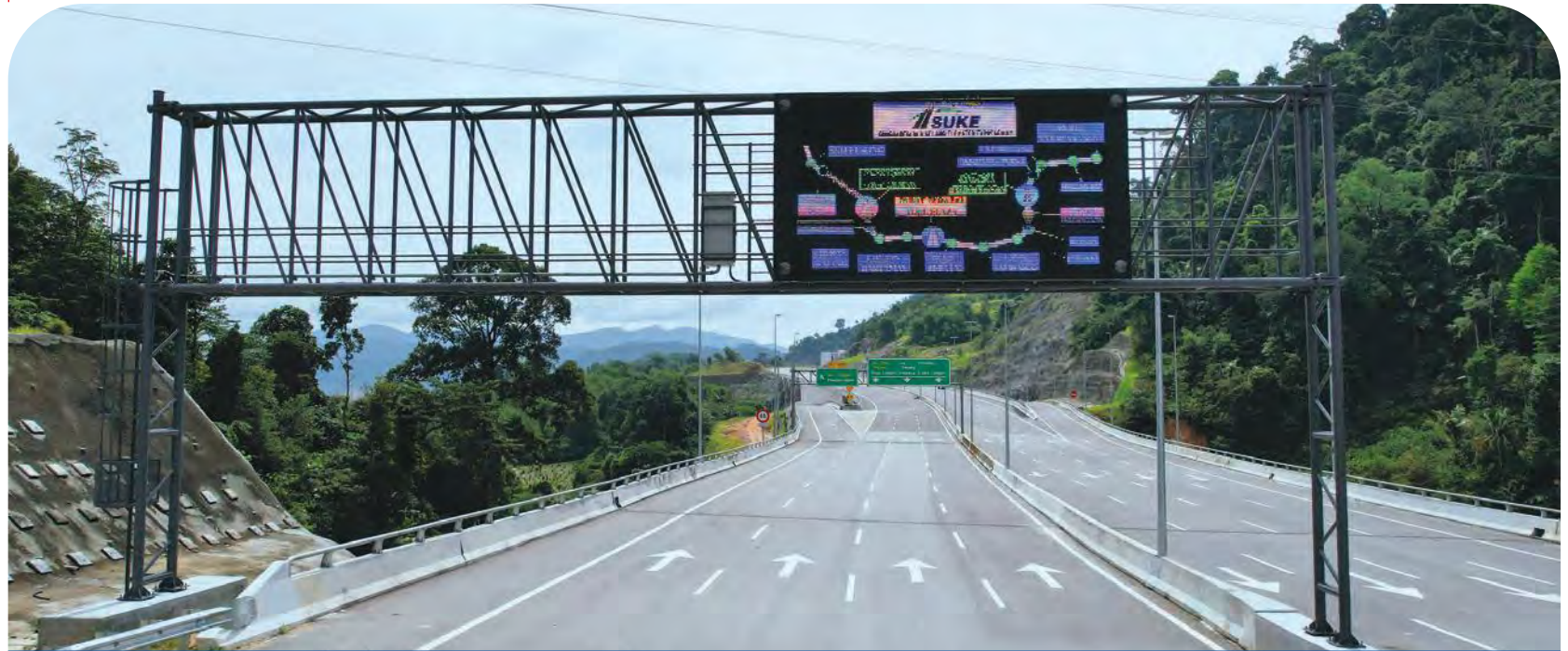
The Variable Message Digital Signage along the SUKE expressway keep road users up-to-date on road conditions.
