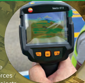
Delamination Spot along Lane 2 (Touch 'n Go) at AKLEH's toll booth.
