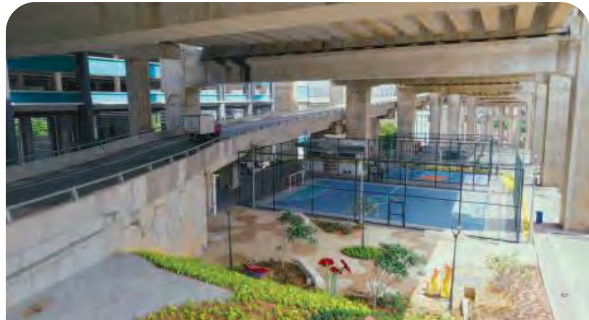
By creating green lungs, we breathe life beneath our highway infrastructures, maximising empty spaces for the recreational benefits of nearby community members and the public.
