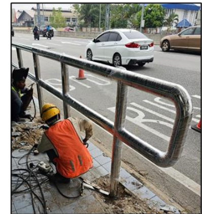
Replacement of Bus Stop Railing at GCE
