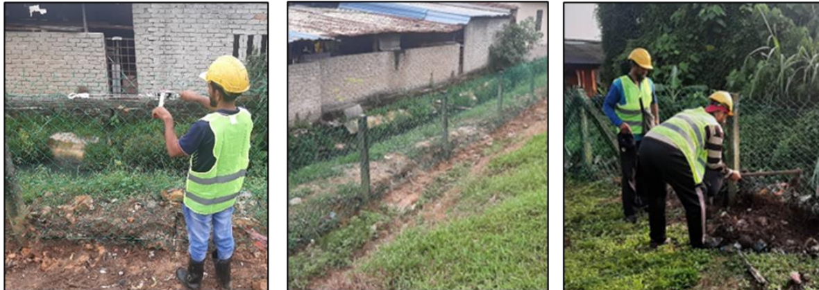
Replacement of R.O.W. Fencing at LKSA
