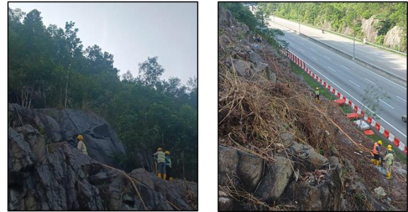
Remedial Work for Soil Slope at GCE
