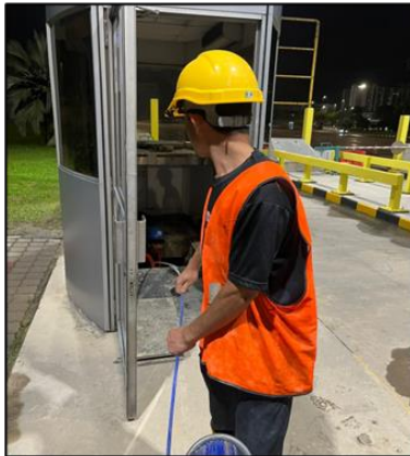
New Power Cable From UPS Room To Toll Booth at SILK
