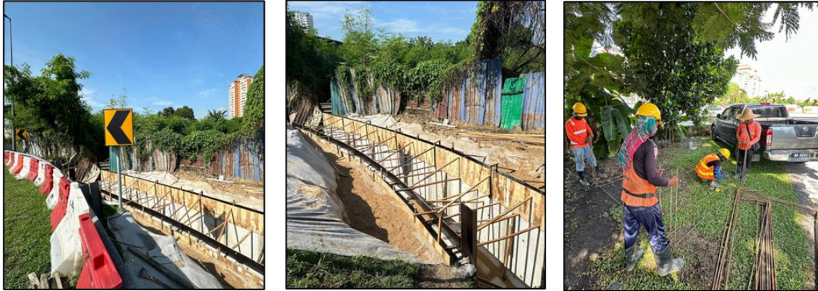
Reinstatement of Damaged Rubble Pitching Slope at GCE
