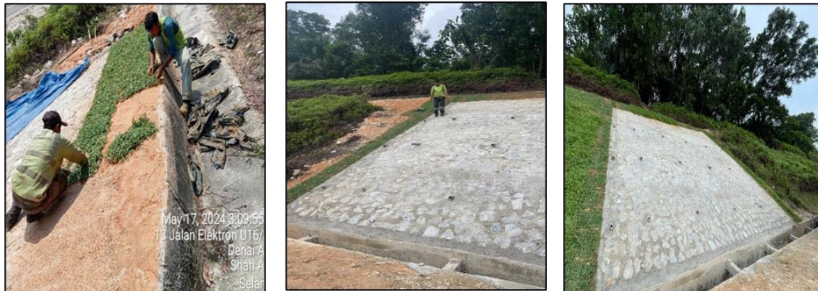
Reinstatement of Damaged Rubble Pitching Slope at GCE
