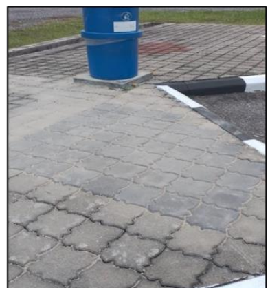
Reinstatement of Damaged Road Kerb & Interlocking at SILK
