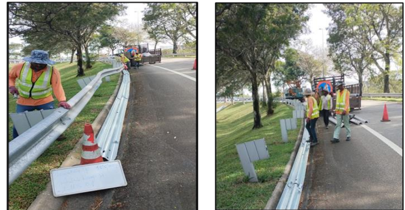
Installation of Guardrail at LKSA
